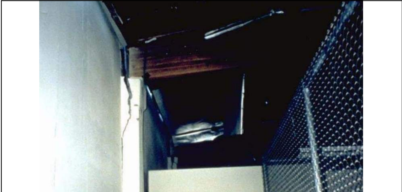
1994 NORTHRIDGE – PILASTER FAILURES
