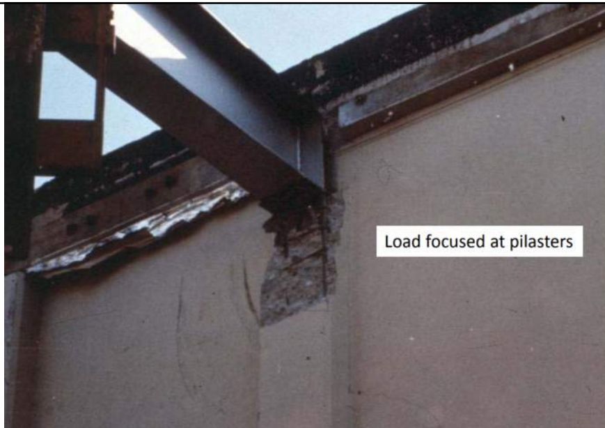
1994 NORTHRIDGE – PILASTER FAILURES
